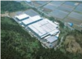
Denyo Fukui Plant, Japan
